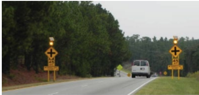
Example of countermeasures on the through approach.
